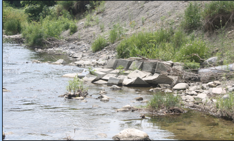
Line 9 Exposed in the Rouge River
